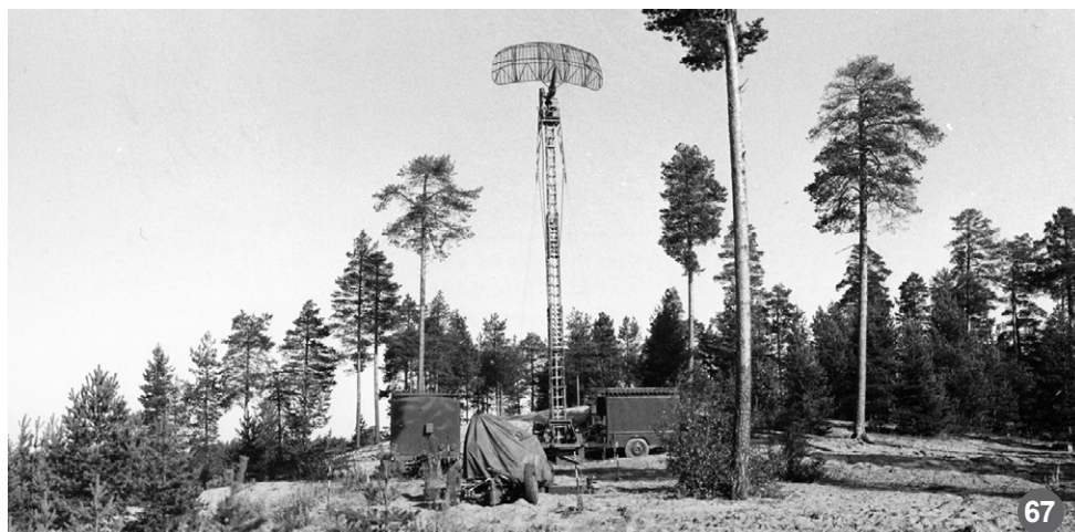
Picture 67: AN TPS observation and target acquisition radar (TEPSU) in Lohtaja. (The Finnish War Museum)
